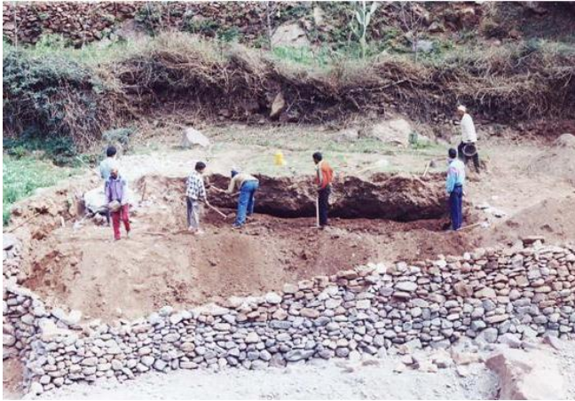
Figure 1 : construction de terrasses
